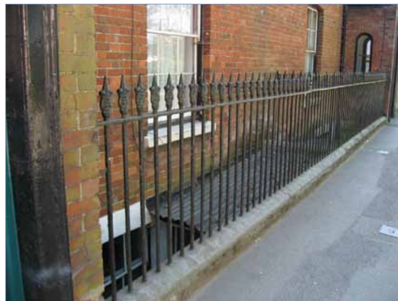
Fig 84 Cast iron railings
