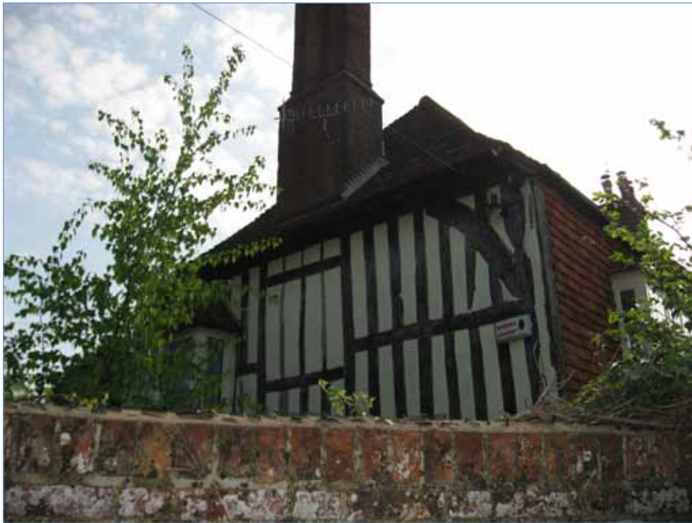
Fig 102 Timber framing, Harnham Road
