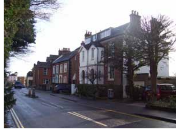
Fig 146 Churchfields Road Villas
